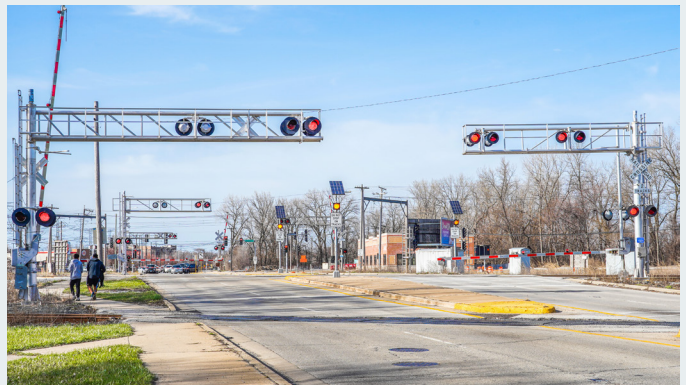
This image shows pedestrians using the existing sidewalk accommodations while downed gates are activated.
